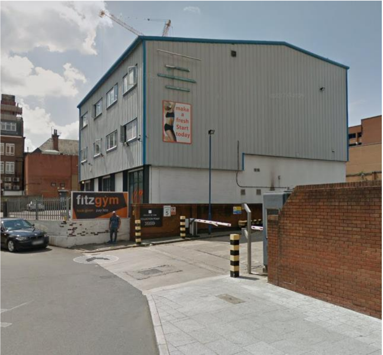
Front/side elevation of Fitz Gym
